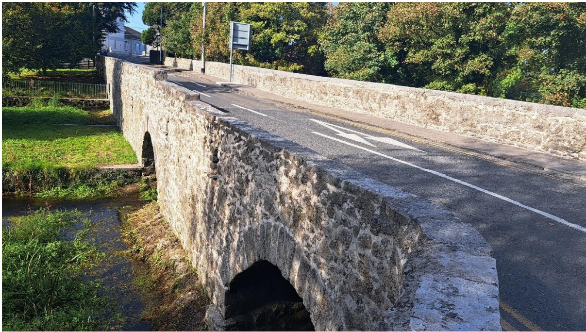
ON THE WEST BRIDGE, BALLINASLOE - COUNTYWIDE BRIDGE REHABILITATION PROGRAMME.
