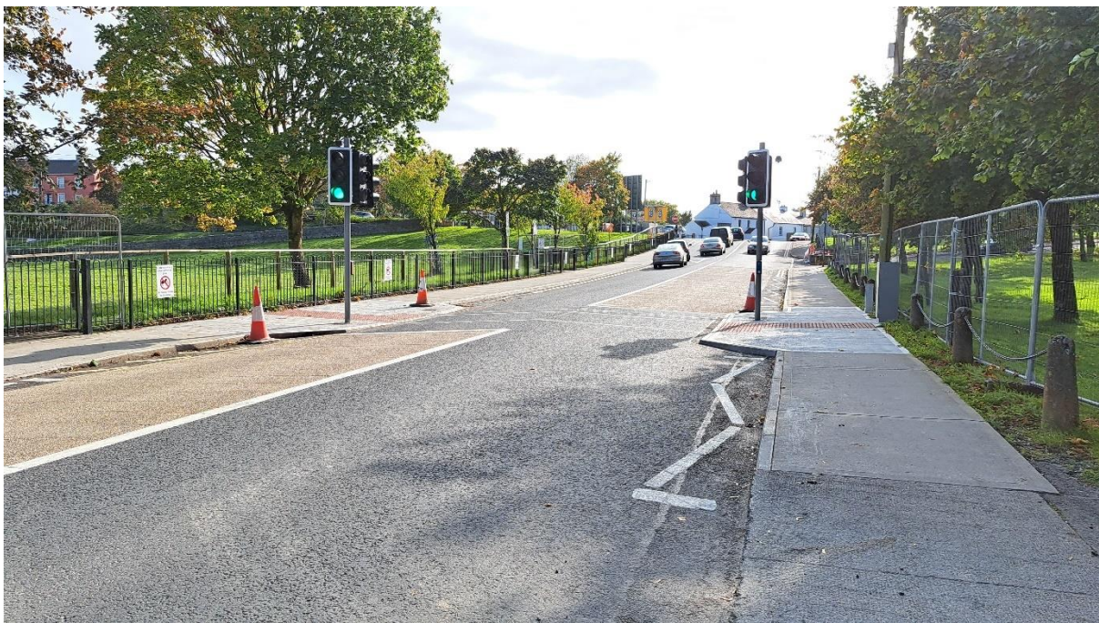
NEW PEDESTRIAN CROSSING INSTALLATION COMPLETED ON HARRIS ROAD, BALLINASLOE.
