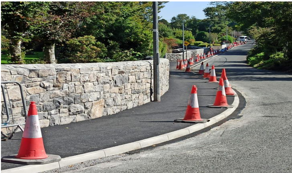
FIG.4 – ANNAGHDOWN FOOTPATH WORKS - COMPLETE
