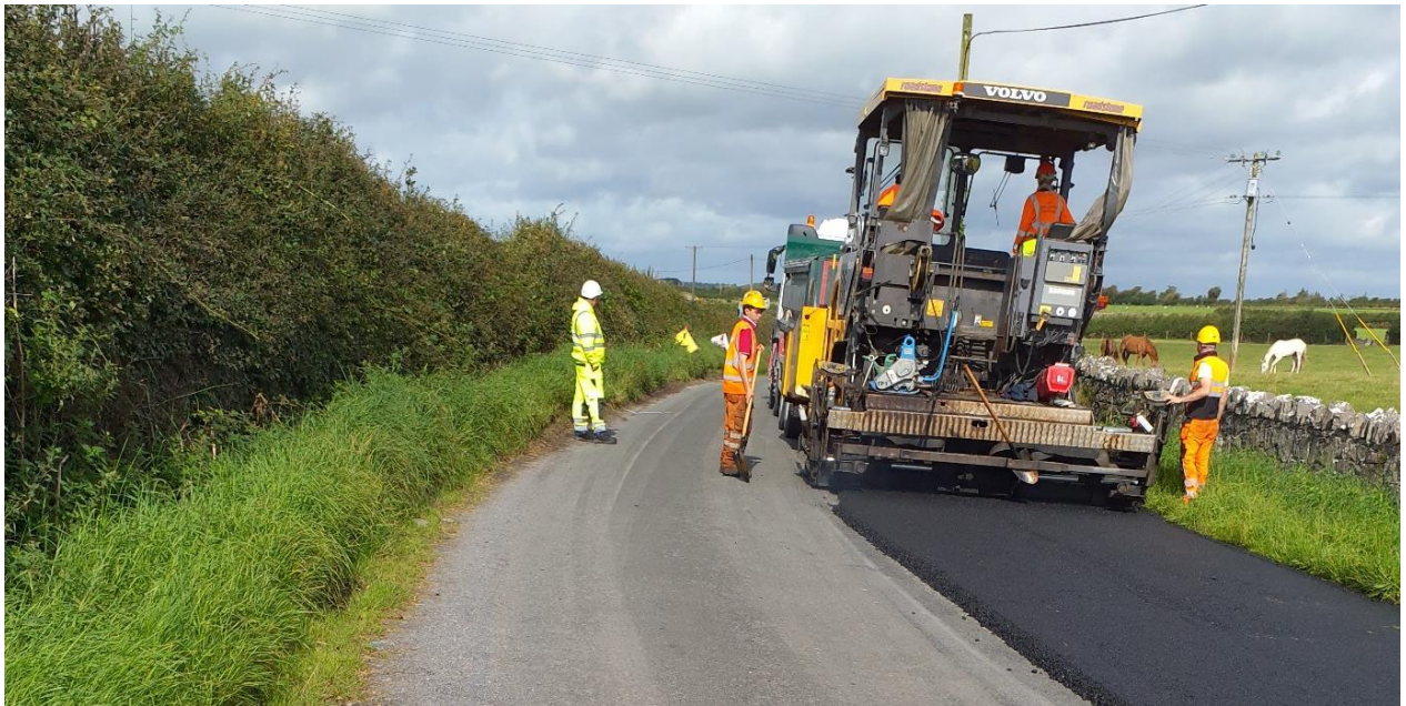
COOLCARTA – STRENGTHENING OVERLAY (RI) – AS WORKS ARE BEING
